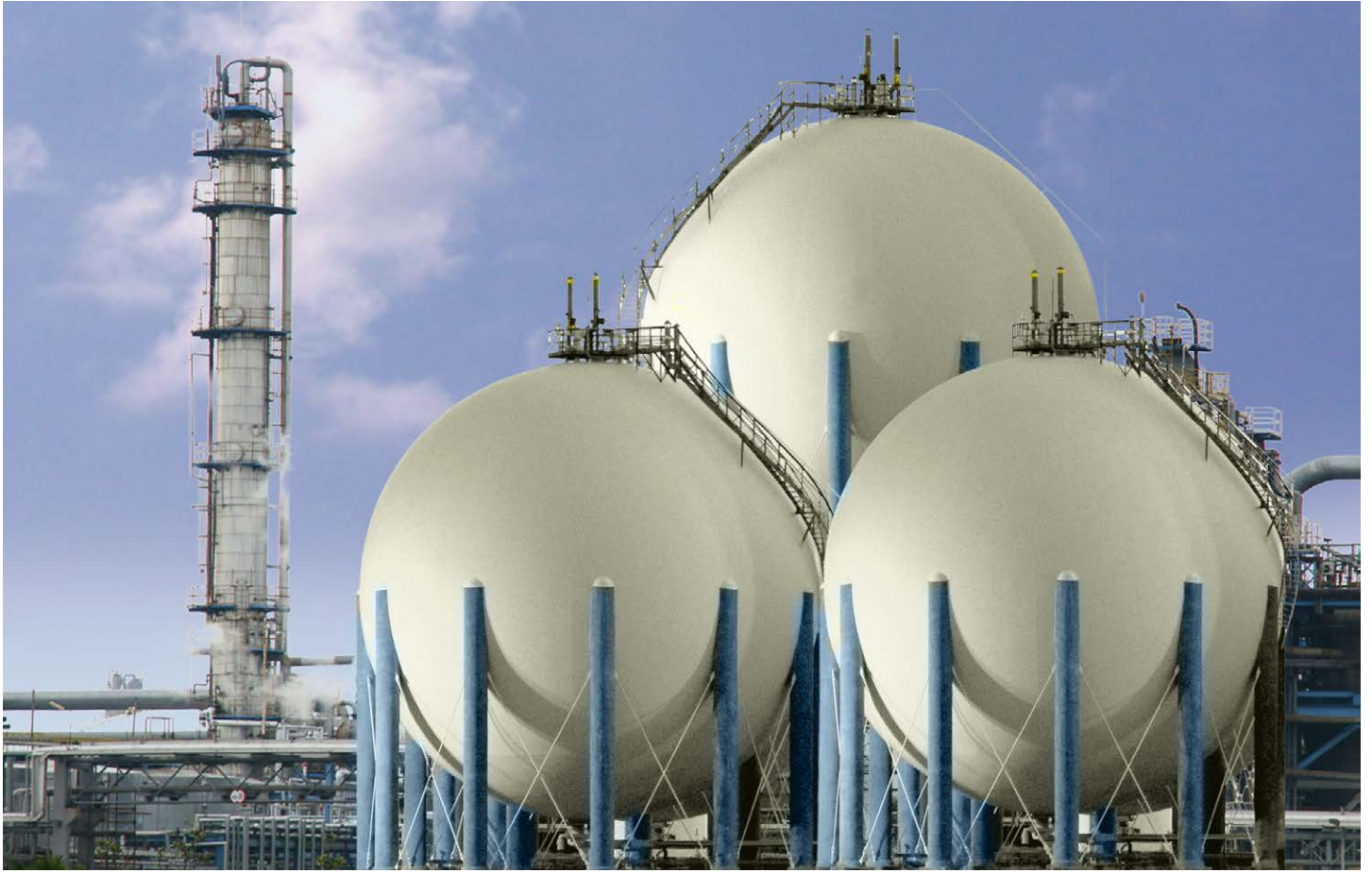
Wire combustion spraying on the inside of chemical and petroleum storage tanks delivers superior, yet cost-effective corrosion resistance.
