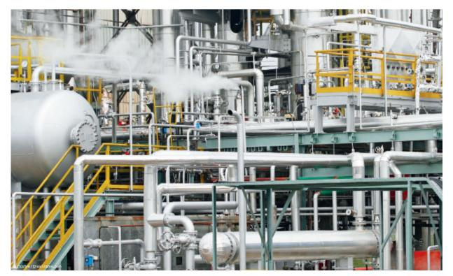
1 Section of a refinery—the piping can be exposed to aggressive fluids under the insulation. environmental damage create entry points for corrosive media. This corrosive media is most often water contaminated with chlorides and sulfates, which gives rise to corrosion under insulation (CUI) [2].
